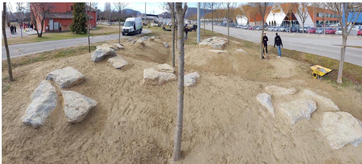
Section building using slabs and blocks of stone and soil to form different slopes - Grade of difficulty: lower and medium.
