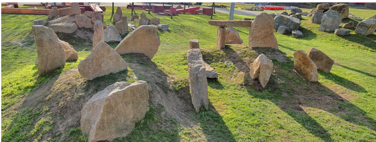
Section using slabs and stone blocks on a soil base and finished with grass - Grade of difficulty: medium and high.
