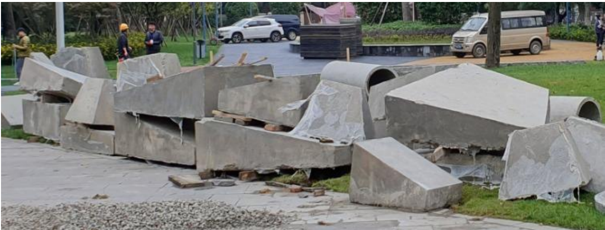
Custom-made concrete pieces before placing them
