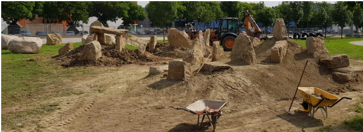
Section building on a soil base with different slopes using slabs and stone blocks.
